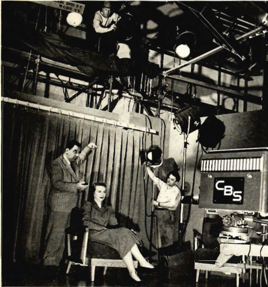
George Stoetzel, CBS' lighting consultant, strives for the desired effect by proper light positioning and angling. A camera check of the image tests the result.
